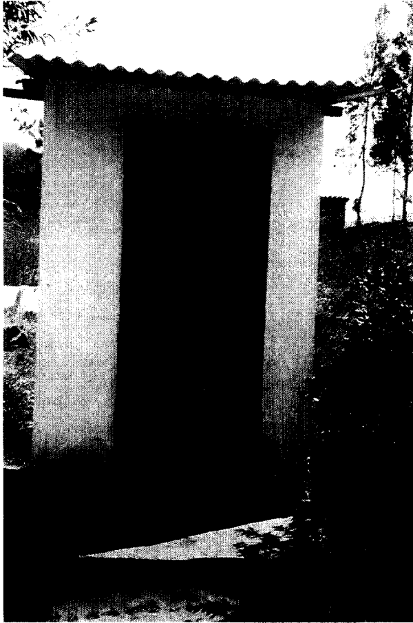
Photo 9. This latrine in Samiapata was constructed through a community microproject.
